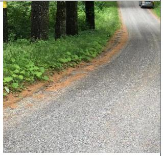
Photo 1: Steep sections of road lack stable ditches.
