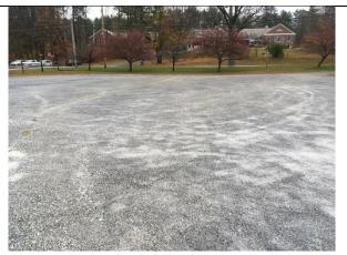
**Photo 1:** Runoff from the gravel parking lot drains **Photo 2:** Gravel parking lot at the library. directly to a catch basin.
