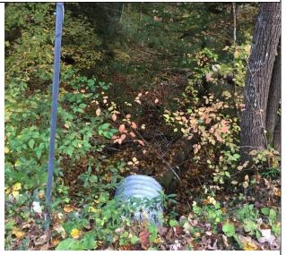
**Photo 1:** Eroded embankment downstream of the culvert outlet.
