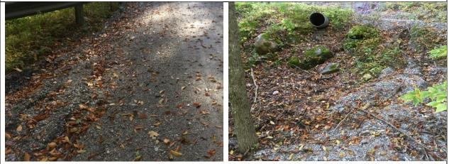
**Photo 1:** Rill erosion from concentrated runoff along the guardrail.
