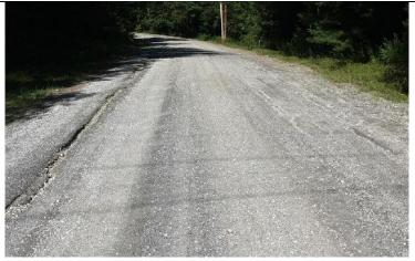
Photo 1: Rill erosion along Wilcox Road observed during road erosion inventories.
