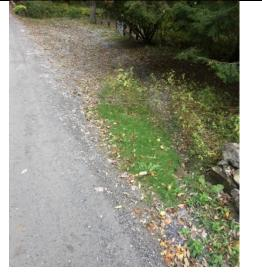
**Photo 1:** Eroded roadway and ditch along West Mountain Inn Road.
