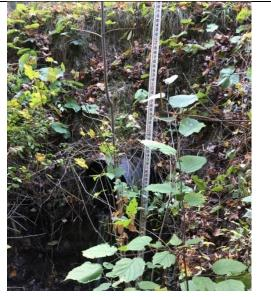
**Photo 2:** Erosion at the culvert outlet.
