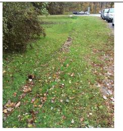
**Photo 1:** Eroded channel along the Fisher **Photo 2:** Existing swale to retrofit. Elementary School Parking Lot.
