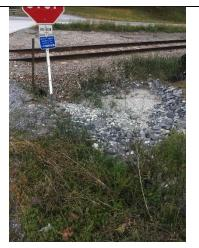
**Photo 1:** Eroded roadside with accumulation of sediment. **Photo 2:** Accumulation of road sediment near a culvert inlet.
