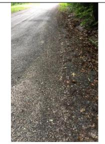
**Photo 2:** Erosion is present on both sides of the road.
