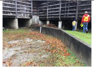
**Photo 1:** Runoff from Munn Drive and Chittenden Drive bypasses a paved berm and flows toward the loading dock during large rain events.
