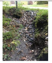
Photo 1: Eroded drainage ditch with accumulation Photo 2: Eroded conveyance along the road of sediment.
