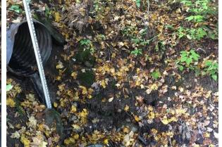
**Photo 1:** Eroded embankment downstream of the culvert outlet.
