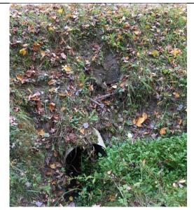
**Photo 1:** Erosion at the culvert inlet header.
