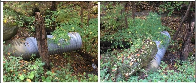
Photo 1: Erosion of the culvert header and outlet.
